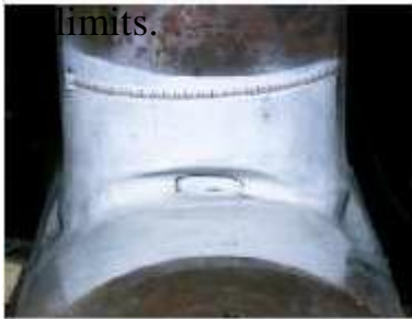
limits. Header – T Weld inspection
