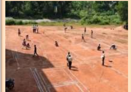
CENTRE LINE MARKING
