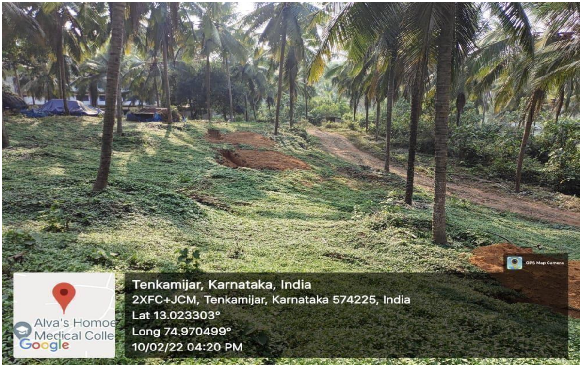
Rain water harvesting percolation pit
