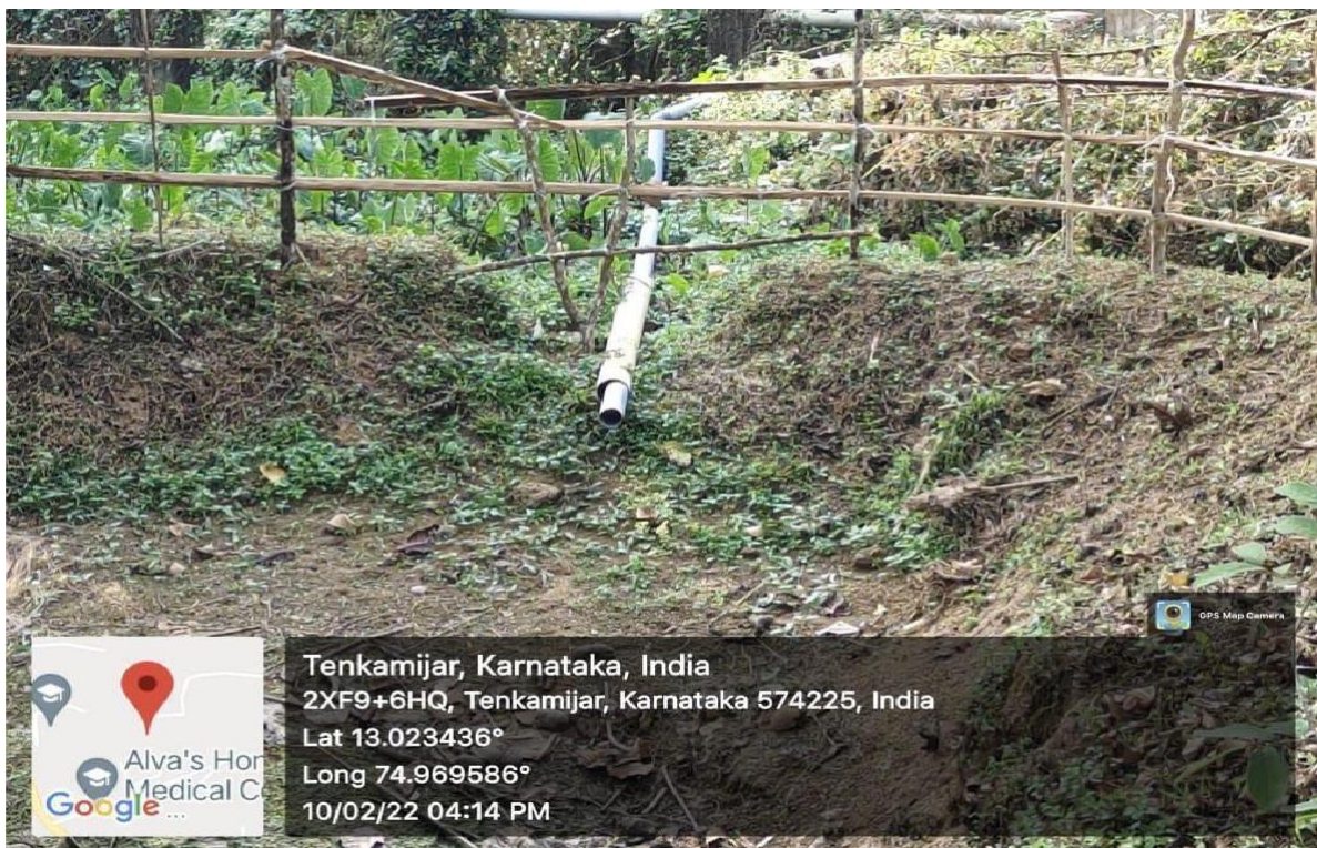
Kumaradhara Hostel D block Rooftop water channelized through Drain pipe to natural pond
