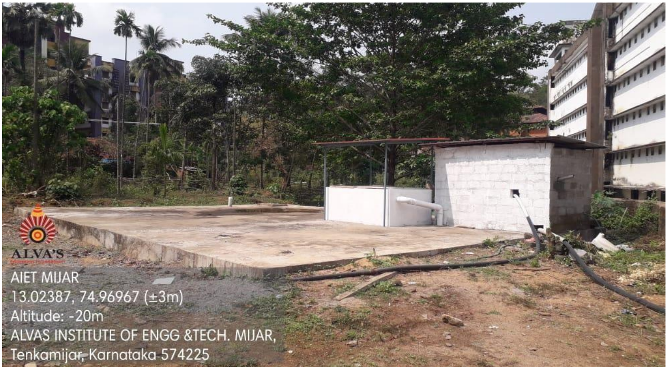
Sewage Collecting Tank of 5 lakh liter
