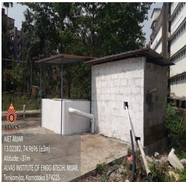
Treatment Chamber of Size 3m x 2m x 1m
